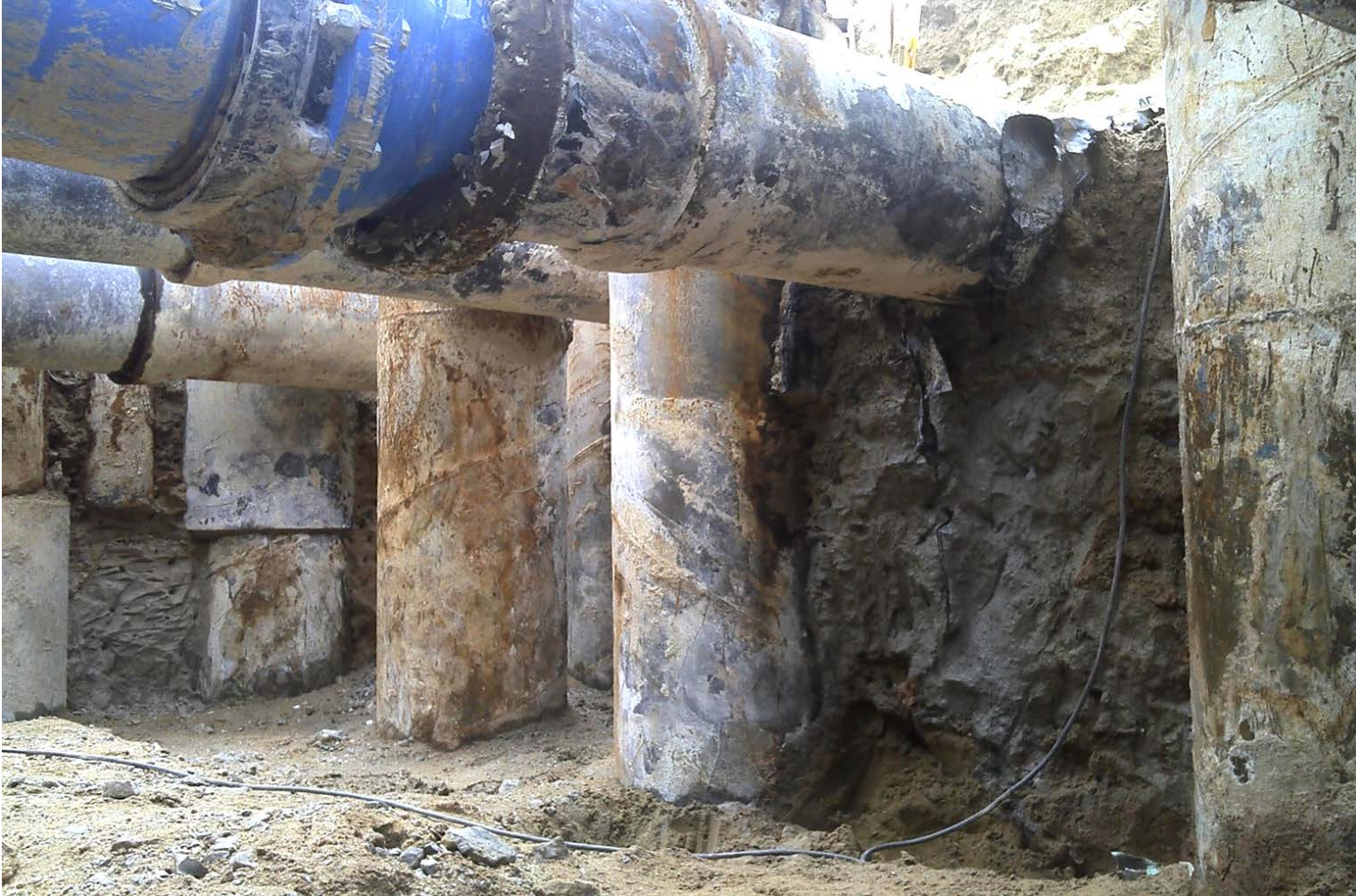
JG columns formed between vertical piles and cooling mains
