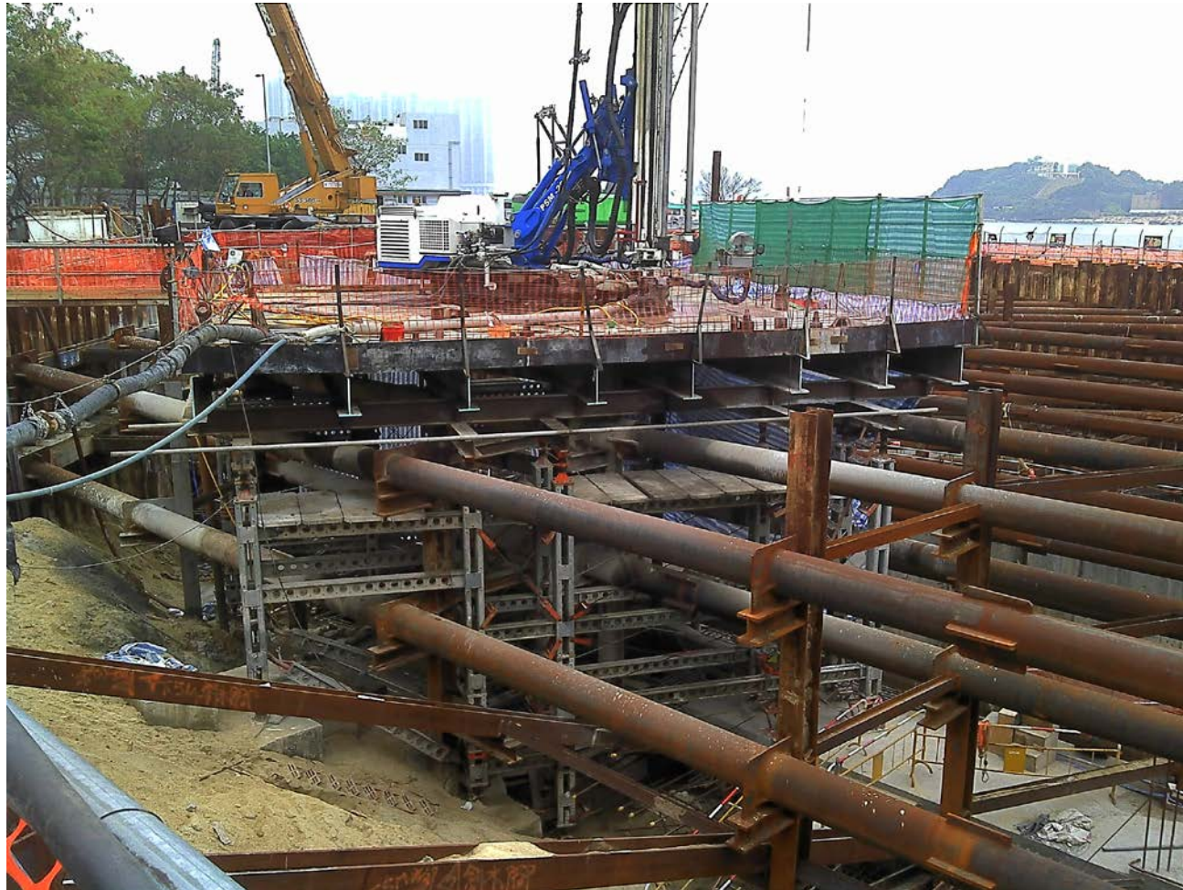
Steel platform erected for supporting the jet grouting rig
